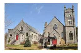
the roof was raised to create a much steeper pitch. At the same time, the square tower was added at the southwest corner, the porch to the west entrance, and the chancel area was also expanded to the east. The Parish Hall was built in 1907 and a new Vestry added in 1965. The walkway between the Parish Hall and the Church was closed in with glass doors in 1985.
